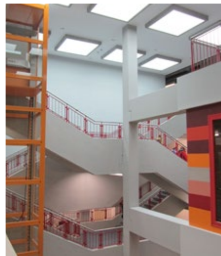
The low energy house standards were adopted in the building and renovation of Sonthofen grammar school.
